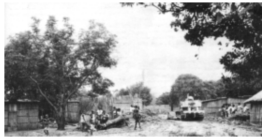
Figure 15. Maxaquene. Opening of access. In: maxaquene, first urban upgrading , page 65.
