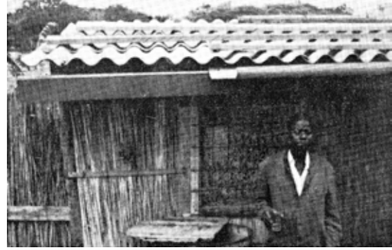
Figure 2. Malhangalene. House of hurdle with covering in fibre-cement foils (Lusalite). In: the Malhangalene Survey , 1977, page. 14.
