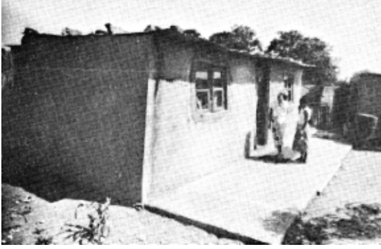
Figure 3. Malhangalene. House with hurdle walls towed with cement and covering with zinc foils. In: the Malhangalene Survey , 1977, page 21.
