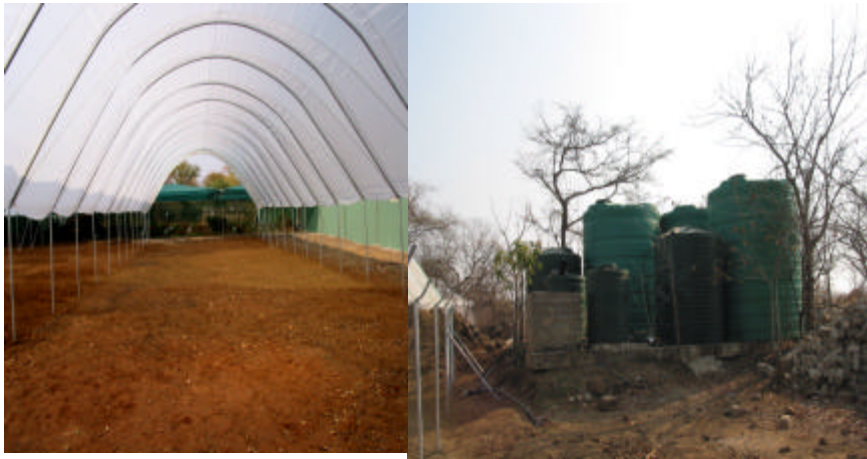
Figure 7: Hydroponics green house and filtration tanks for the vulnerable groups' project in Livingstone.
