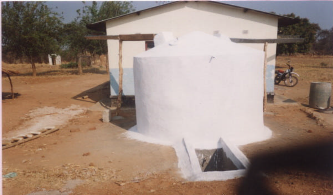
Figure 5b: Construction of Ferro-cement Tank at Simbulo Basic School Choma.
