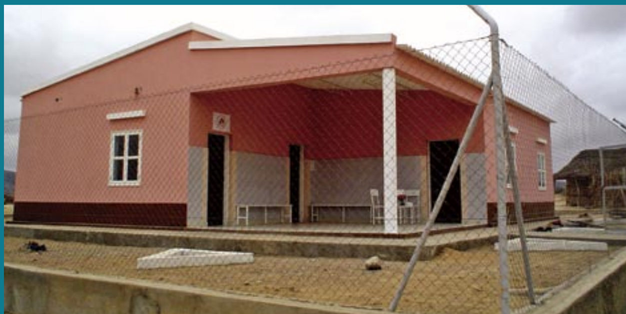
A HEALTH POST CONSTRUCTED BY FAS
