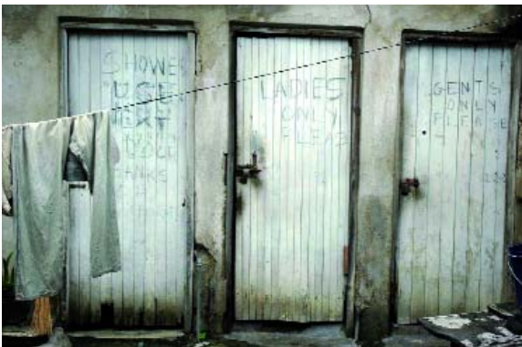
Above A toilet block in Dar es Salaam, Tanzania.
