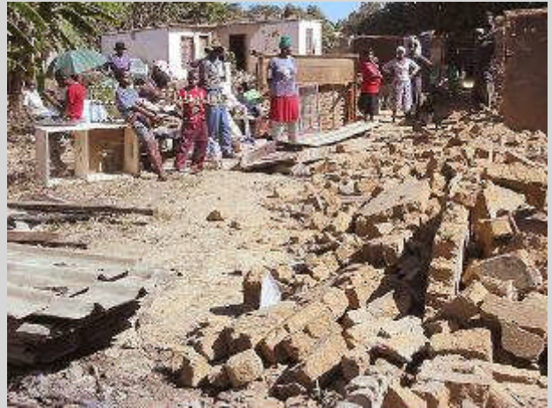
Family Demolishes own house in Epworth, Harare.
